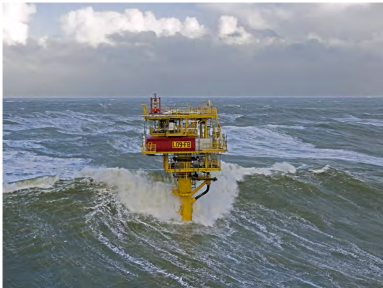
"L9" platform in the Southern North Sea.
